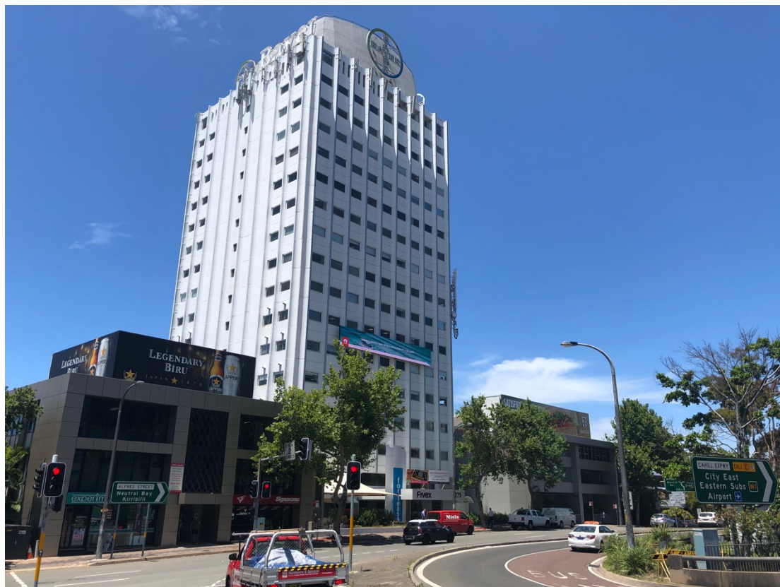
Figure 5 – Built form along Alfred Street Source: Grimshaw
